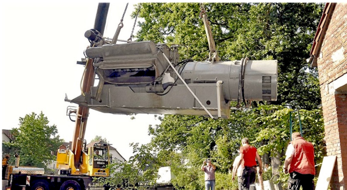
Abb. 4: Notstromaggregat
